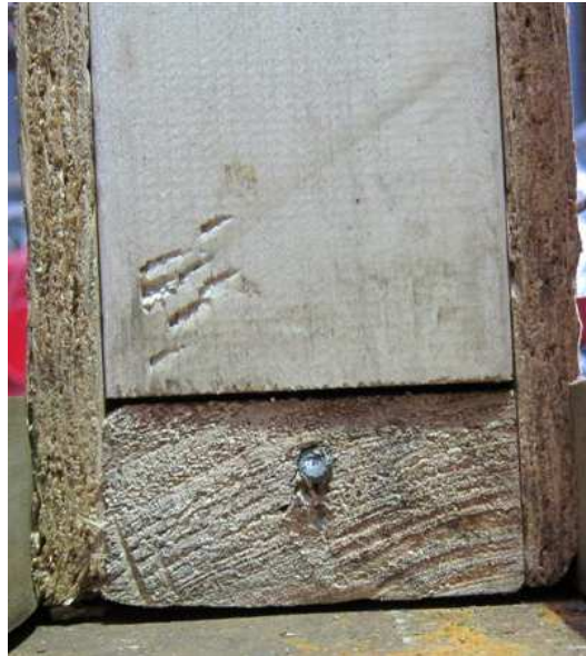
Figure 14: Racking test specimen showing where 8mm coach bolt has sheared in wall base plate after 20mm racking deflection
